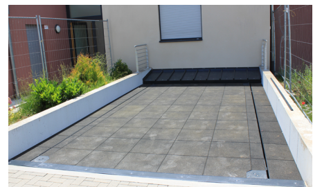
Rubber covering in stone structure (3 cm thick)
