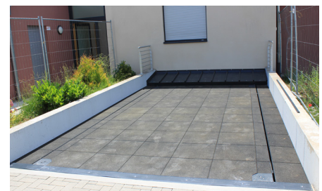
Rubber covering in stone structure (3 cm thick)
