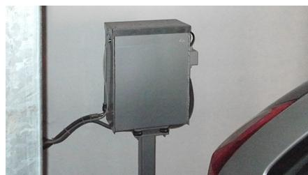
With hydraulic piping and cabling to the system. (The under oil unit is not noisy thanks to the motor-pumps-combination that absorbs sound and insulates from noise).
