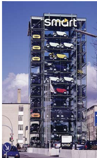
SMART TOWER SIZE XXL Special project planning for smart in Hamburg (Germany), storing and presenting of 86 smart fortwo vehicles on a total height of 24 meters
